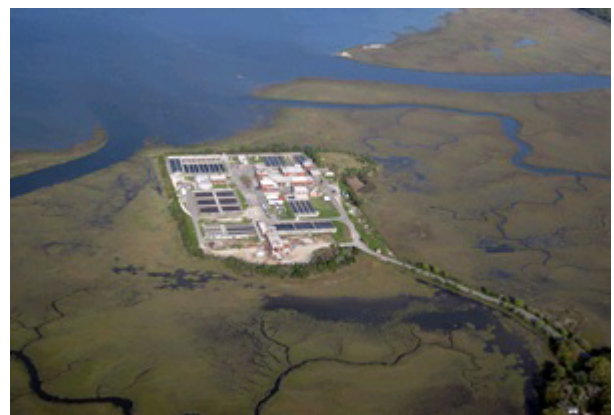
Plum Island Wastewater Treatment Plant in Charleston, SC, one of the study areas, is shown above.
